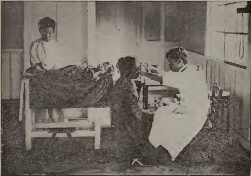
MAKING REPAIRS IN HANABATAKE DISPENSARY
